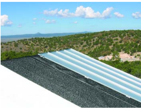
Enkamat creates a drainage plane by spacing the roof from the roof sheathing. 1
