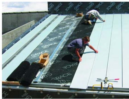
Workers walk directly on mat without damaging product or weather barrier. 1
