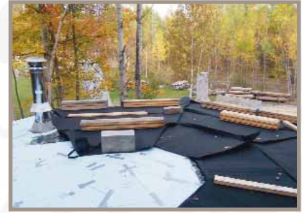
Trapezoidal pieces of Enkadrain 3615 cover the octagonal roof.
