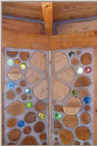
Interior cordwood masonry wall detail.
