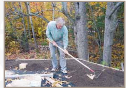
Rob Roy spreads topsoil (400 pails in all) over Enkadrain.
