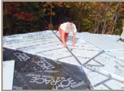
Jaki Roy tapes the Styrofoam together over the waterproofing membrane.
