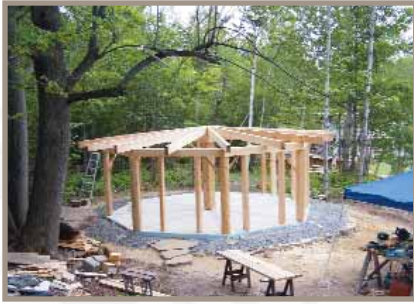
The octagonal post and beam timber frame.
