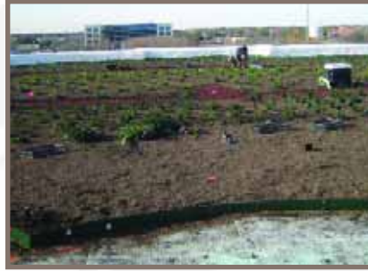
Specially formulated planting medium and native plants are chosen for the project.
